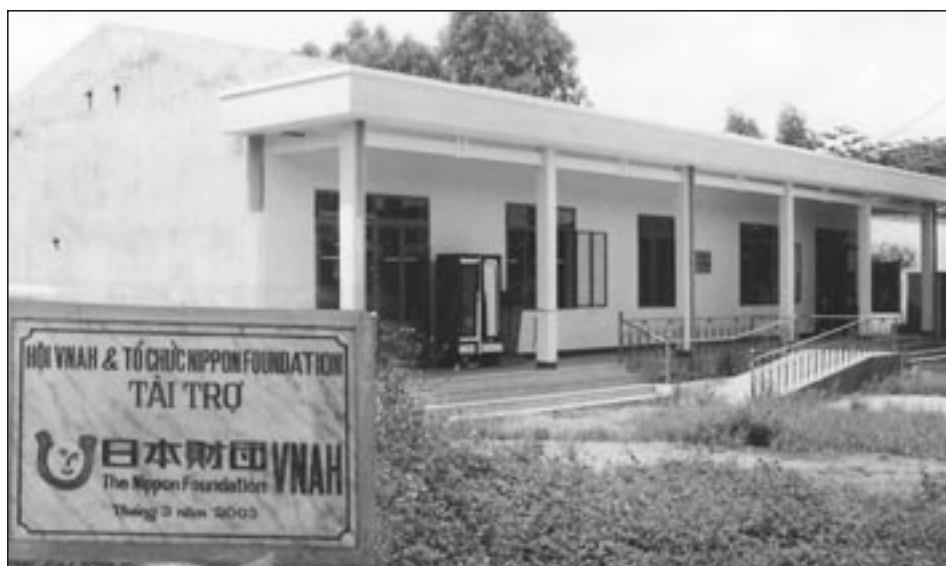
This new building was completed in March 2003 with the help of funding received from the Nippon Foundation. It is used for vocational training classes in Lien Chieu Town in the suburb of Danang City.
