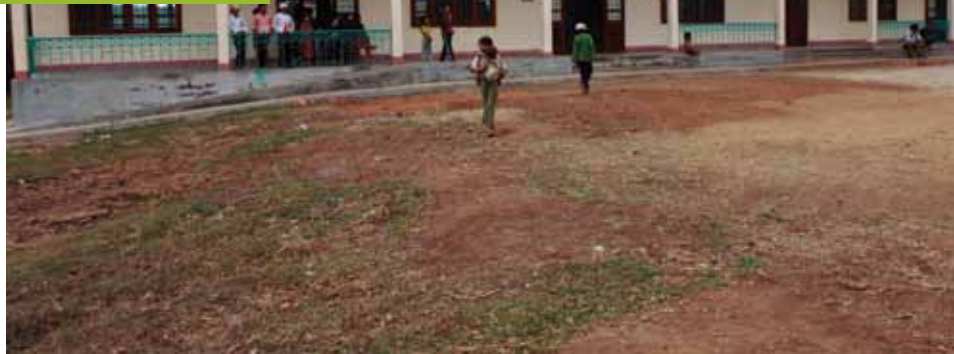
A new 3-room school replaces the old school below.
